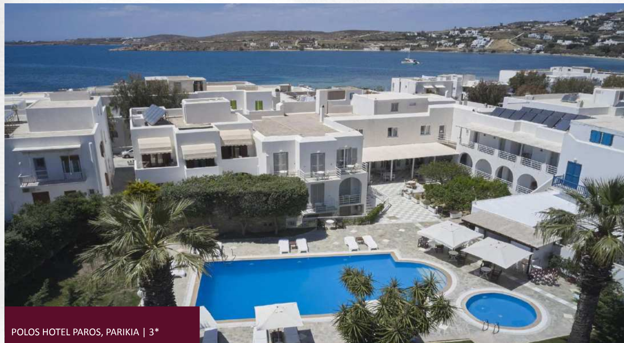
SAN ANTONIO SUMMER HOUSE, PISO LIVADI | 3 KEYS
